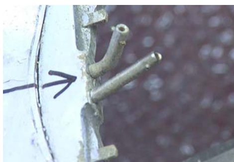
Figure 107: Aft hinge & stop pins, (looking from outside to inside)
