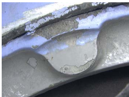
Figure 191: Upper stop pad; paint chipped.
