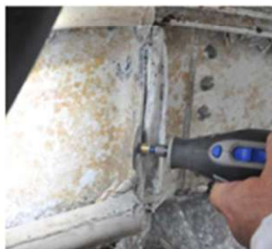
Cutting off joint moulding to check repair
