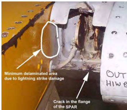
Fig. 7a The damage to the main beam flange at the outboard hinge
