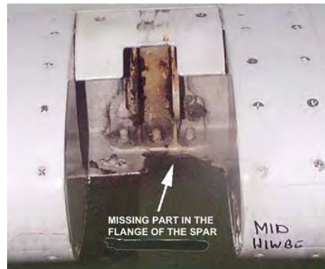
Fig. 7b The damage to the main beam flange at the centre hinge
