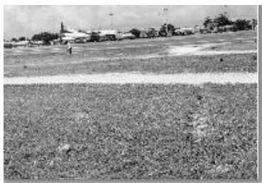
Fig 9. Wheel marks on the unpaved surface.
