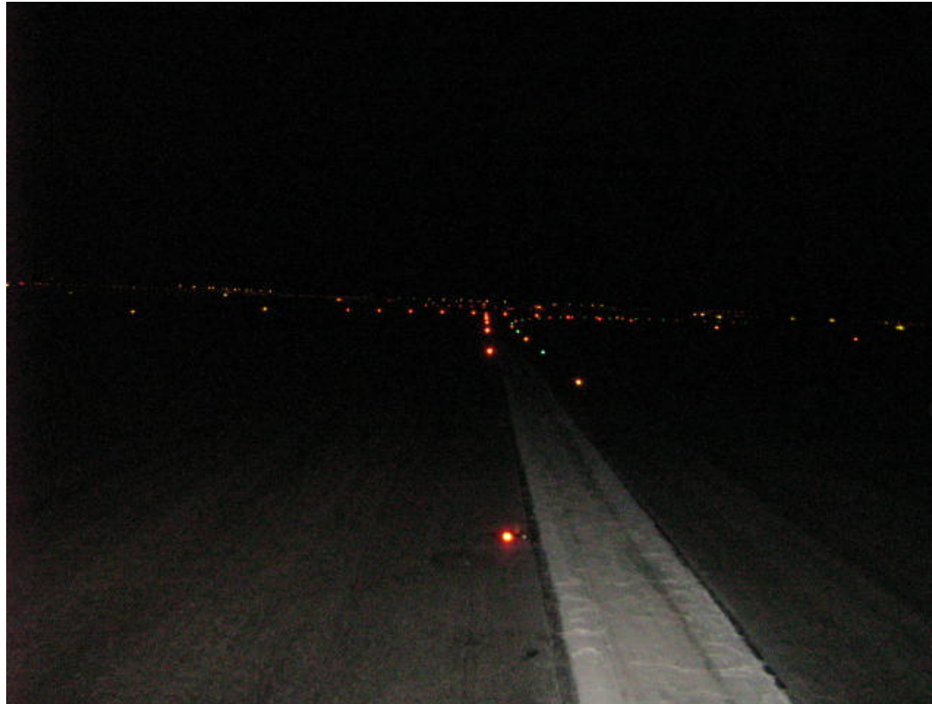
Figure 4. Distance-coded runway centre line lights and runway end lights near the shortened end of Runway 20C
