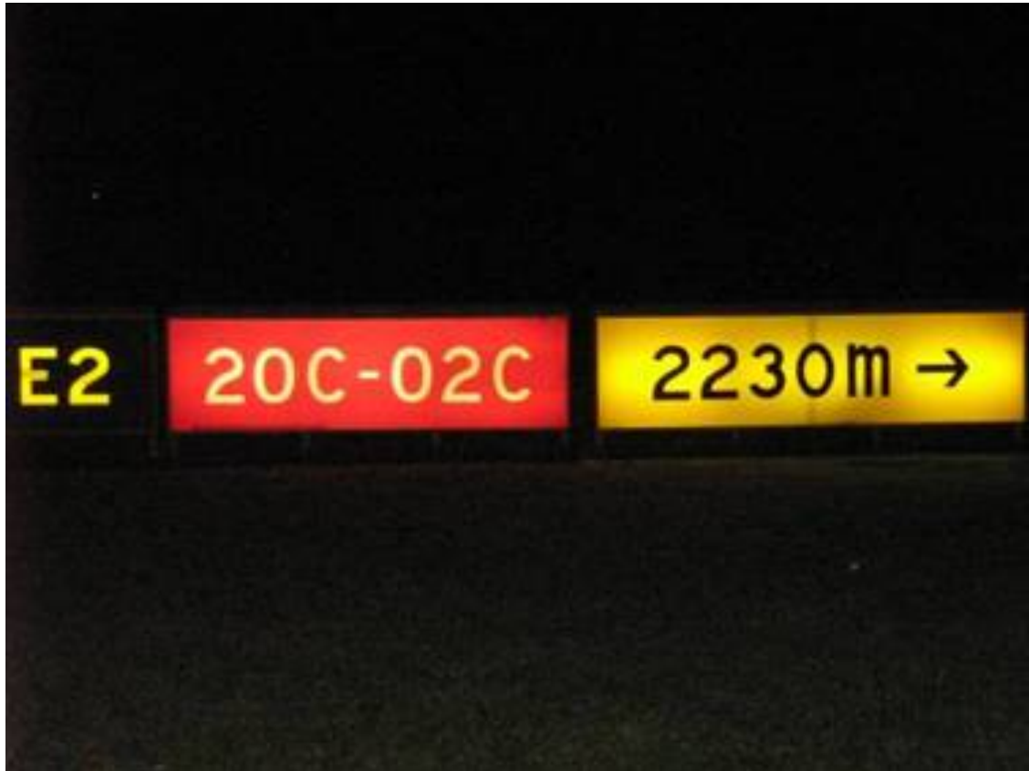
Figure 6. Guidance sign at E2 taxiway holding position after the original inscription panel showing 3850 m was replaced with one showing 2230 m
