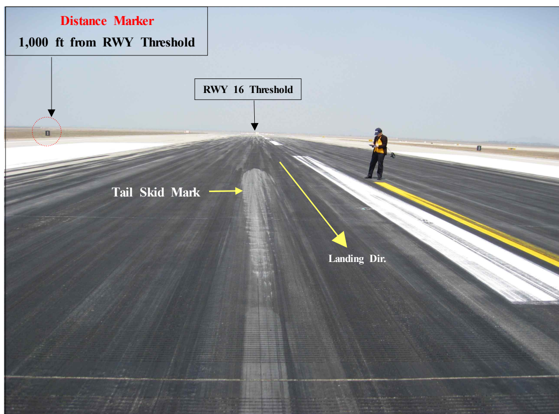
[Figure 7] Tail Skid Mark on Runway
