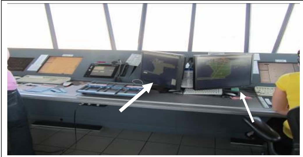
Figure 43 shows positioning of the A-SMGCS Traffic Context screen at FAOR Tower
