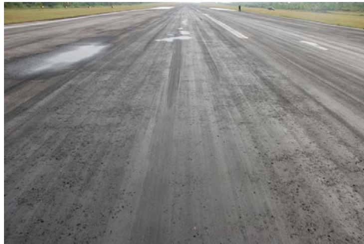
Figure 3: Rubber deposit on the touchdown zone runway 18.
