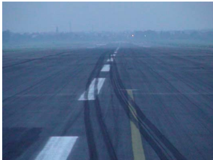
Figure 6: Tire mark on runway close to taxi way D
