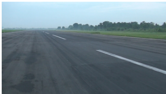
Figure 6: Tire mark on runway close to taxi way D
